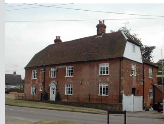
Traditional lime mortar repairs
