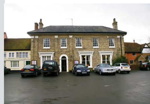
Replacement Georgian brick facade of Hayes House
